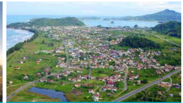
Aceh Road/Bridge Reconstruction | Banda Aceh, Indonesia USD $282 Million | Design and Construction Management
