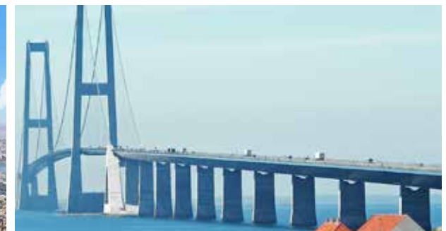
Great Belt Eastern Bridge | Storebælt, Denmark USD $600 Million | Construction Management
