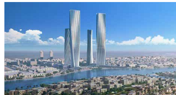
Lusail Development Project | Doha, Qatar | USD $5.5 Billion Program Management and Construction Management
