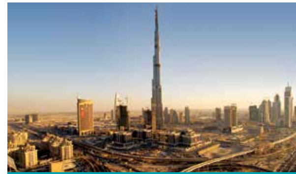
Dubai Metro | Dubai, UAE | USD $8 Billion Program Management and Construction Management
